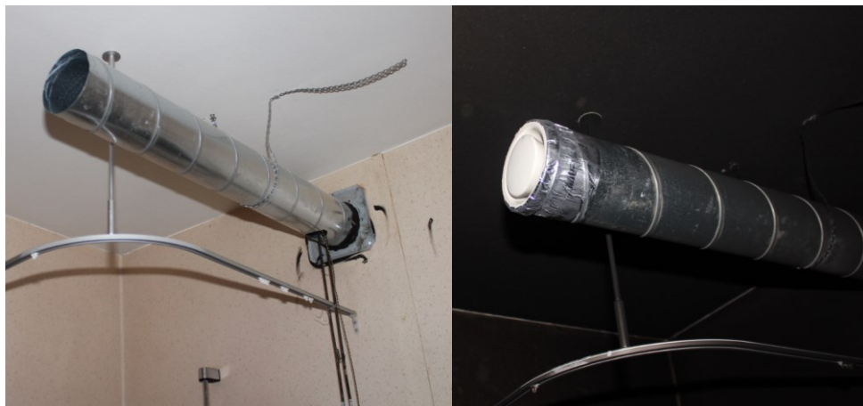
Figure 9: Exhaust ducts configurations – Open condition (left), Normal condition (right)
